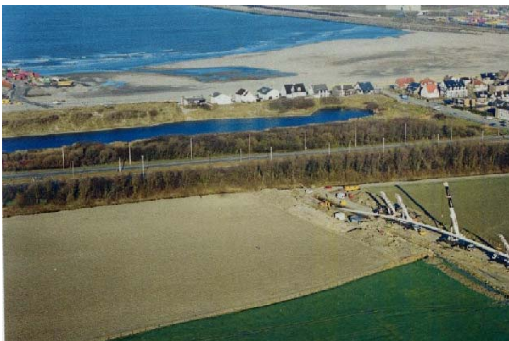
Figure 8: Drilling under the Freshwater Lake and Dunes at Zeebrugge
